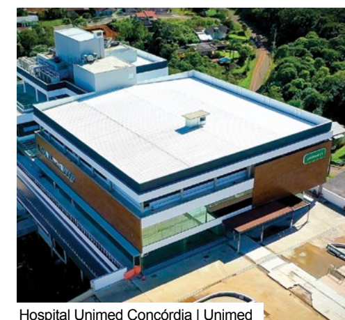
Hospital Unimed Concórdia | Unimed
